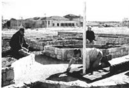
Laying first bricks
