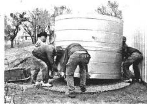
Setting the tank
